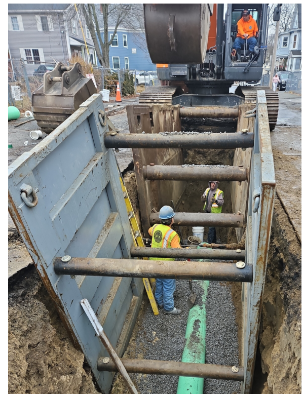
Sewer main installation on Tenney Street
