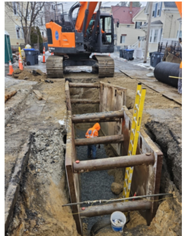
Drain main installation on Tenney Street
