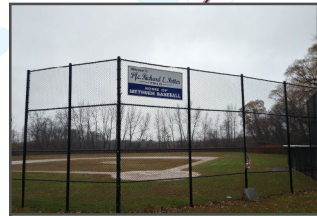
Pelham St Ballfield lighting & improvements
