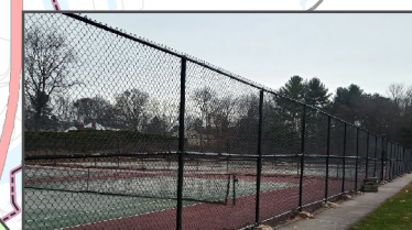
MHS tennis courts & baseball field resurfacing
